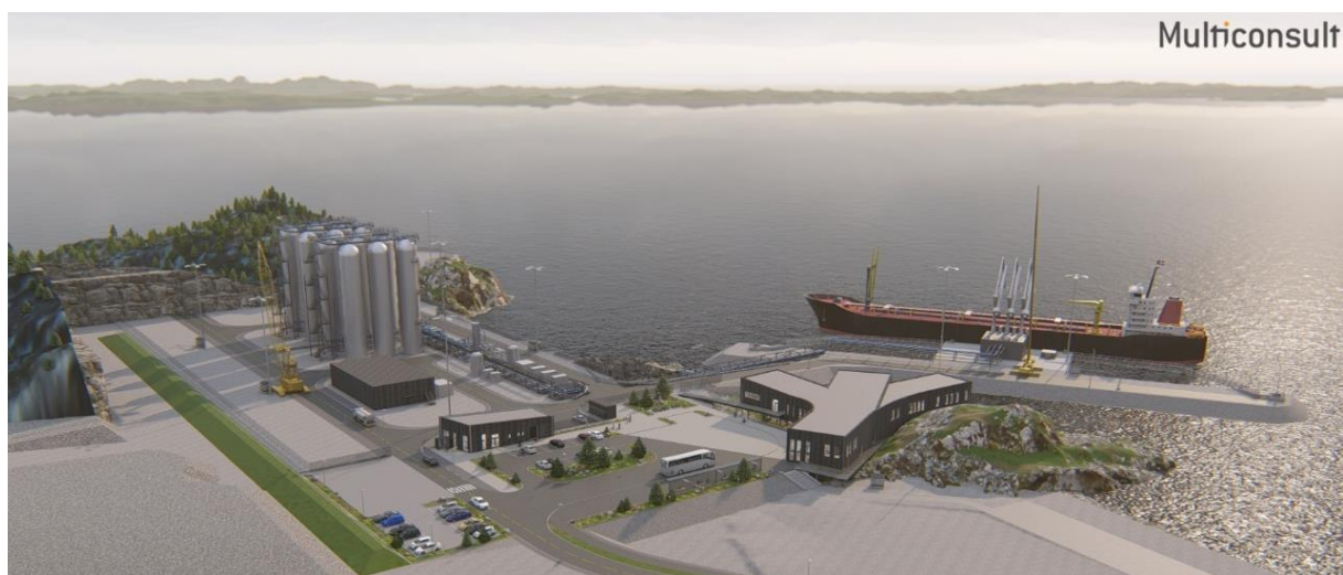
Figure 3-9 Illustration of receiving facility with administration building and visiting area on the right, warehouse building by the car park and parts of the tanks with power grid station to the left. Viewed toward the southeast. Illustration: Multiconsult.
