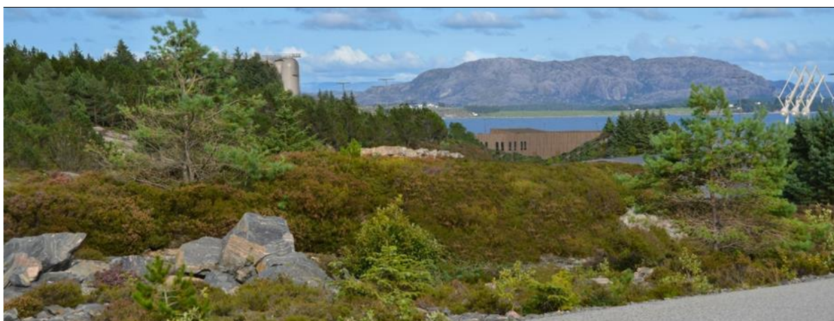
Figure 5-13 Photomontage 1, showing the tanks to the left, the administration building in the centre and the offloading arms to the right. Seen from the access road (Ljøsøyvegen) towards the industrial area by Hjeltefjorden. Illustration: Rambøll.
